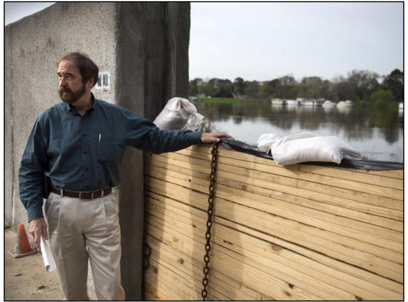
Inspecting the flood wall in downtown Monroe, La., March 16, 2016
