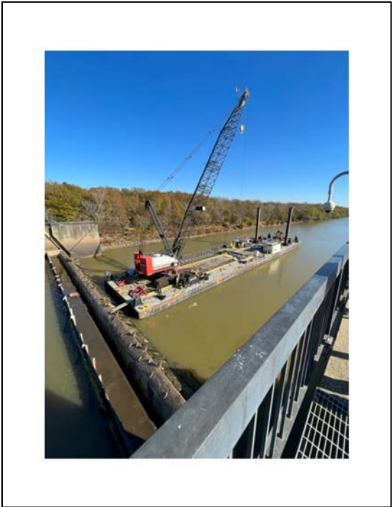
Picture above of the removal of the leaking hinged crest gate from the Thatcher Lock and Dam. A “Poiree needle system” supported by thick steel I-beams is in place until a replacement hinged crest gate arrives.
