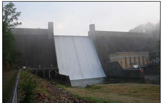
Flood waters flow over the spillway for the first time since 1968.
